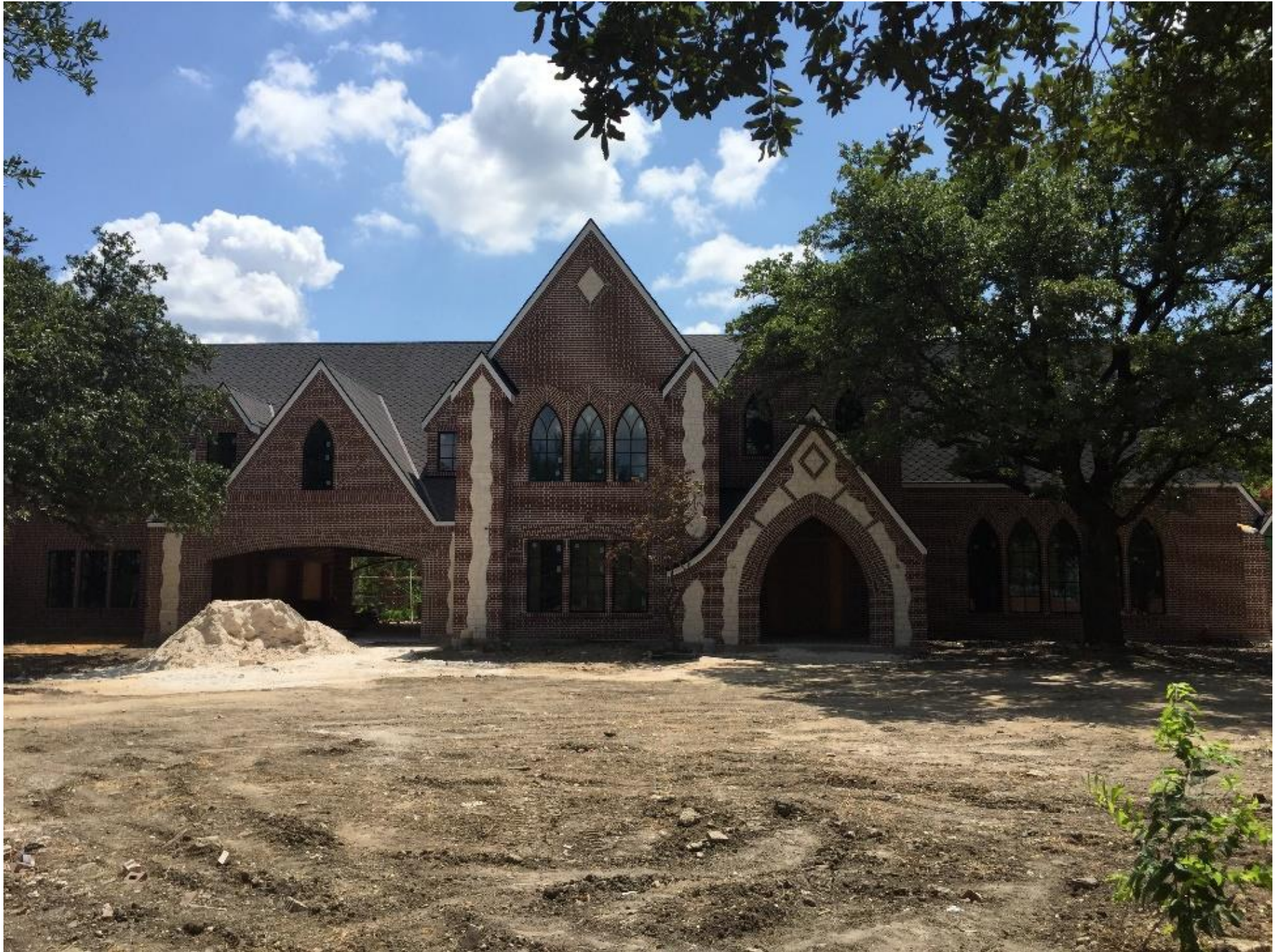
11,000 s.f. residence in north Dallas 2016—2018. Under construction.
