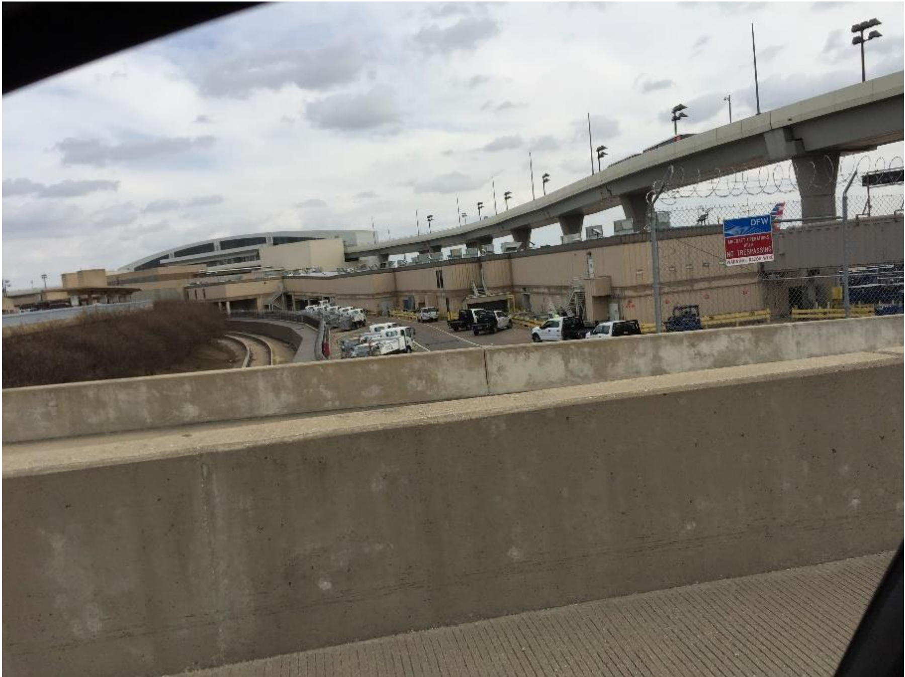
1 of 7 DFW Airport Skylink stations. I managed the design & engineering process for prototype.
