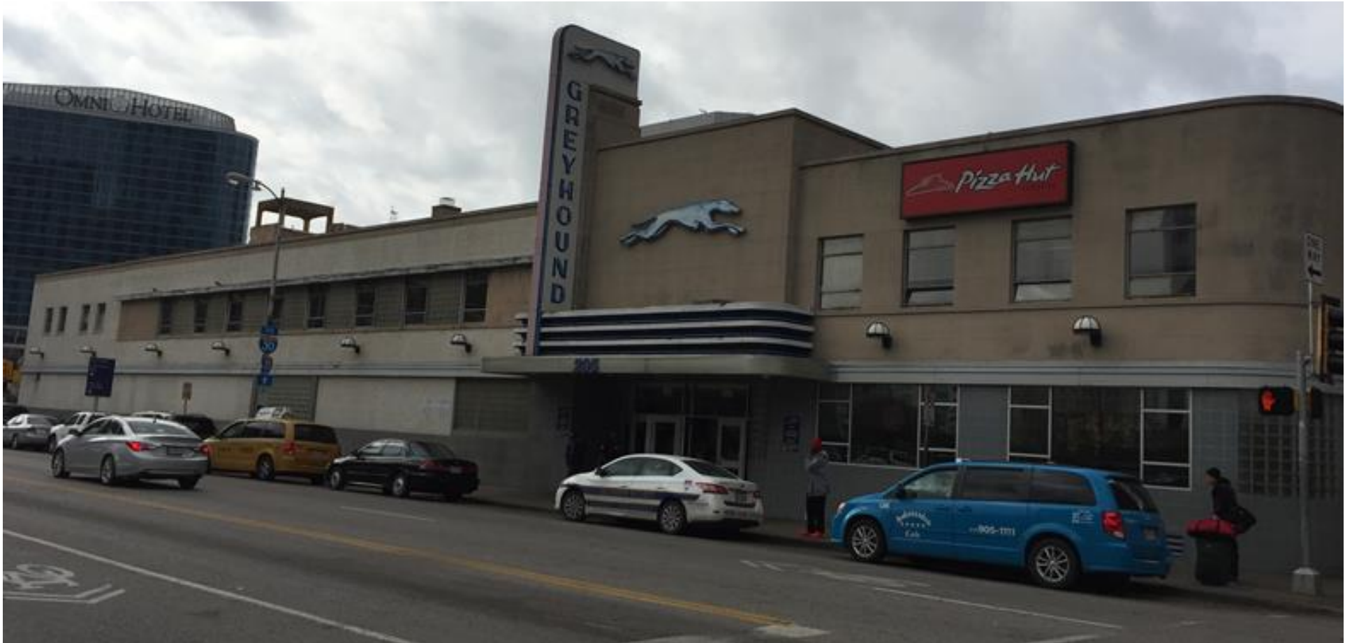
I managed entire design and construction project of Dallas Greyhound Terminal Renovation.
